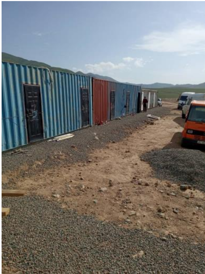
Figure 14: The area of the additional construction camp (km 106+300)
