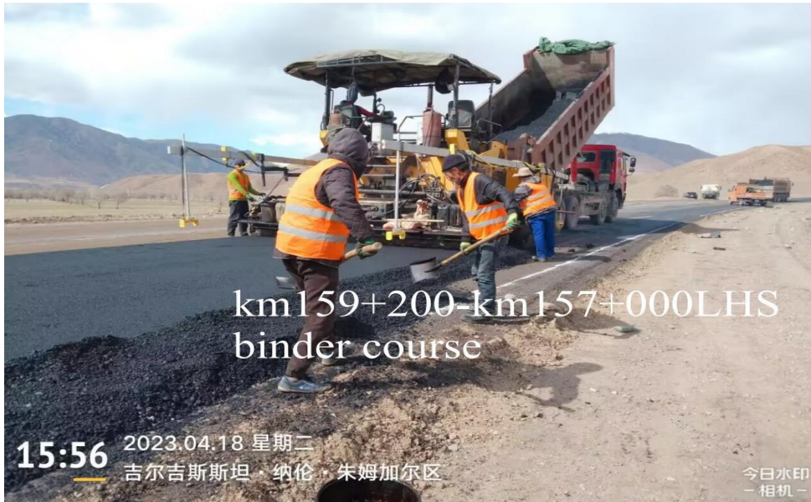
Figure 15: Constuction activities on project road
